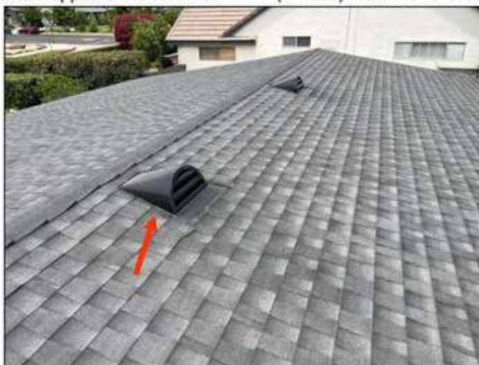
(roof vent AS) Roof appears to be properly vented, vents are installed appears serviceable.
