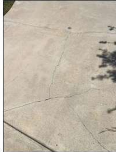
Driveway had common cracks *, Appears serviceable.
