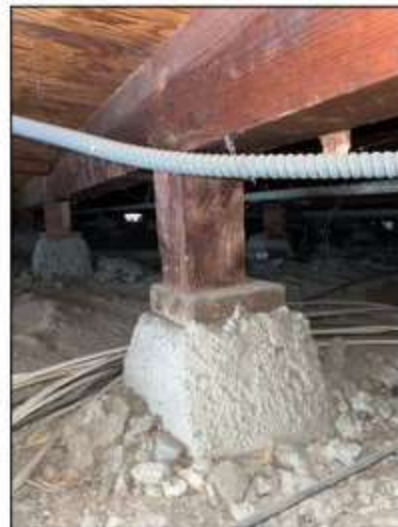
Raised foundation support is post and pier.
