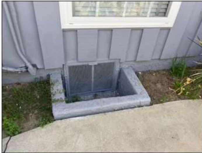
(foundation access W) Foundation crawl space access located at exterior west side.
