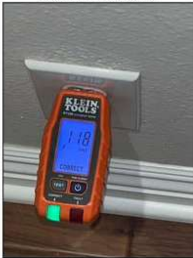
A fair of number of electrical outlets were tested at the time of the inspection for correct voltage, the electrical outlets tested at 120 Volts which appears serviceable.
