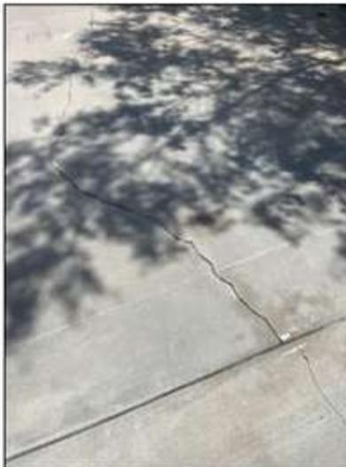
Driveway had common cracks *, Appears serviceable.
