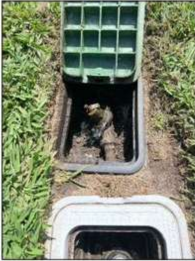
Pressure regulator installed at front of main water supply at meter area.
