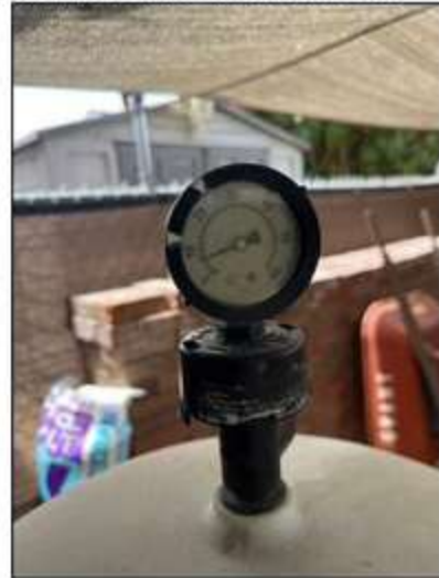
Filter canister pressure gauge and relief valve installed, appears serviceable.
