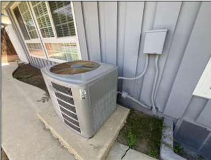
(W) HVAC Compressor located at: Exterior south side, see notes below for other issues noted.
