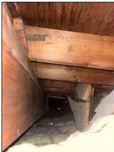
Attic structure is conventional wood framing 2x4 ceiling joist and 2x4 roof rafters, wood panel roof. Attic structure is conventional wood framing 2x4 ceiling joist and 2x4 roof rafters, wood panel roof.
