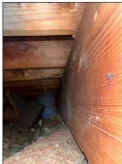
Attic structure is conventional wood framing 2x4 ceiling joist and 2x4 roof rafters, wood panel roof. Attic structure is conventional wood framing 2x4 ceiling joist and 2x4 roof rafters, wood panel roof.
