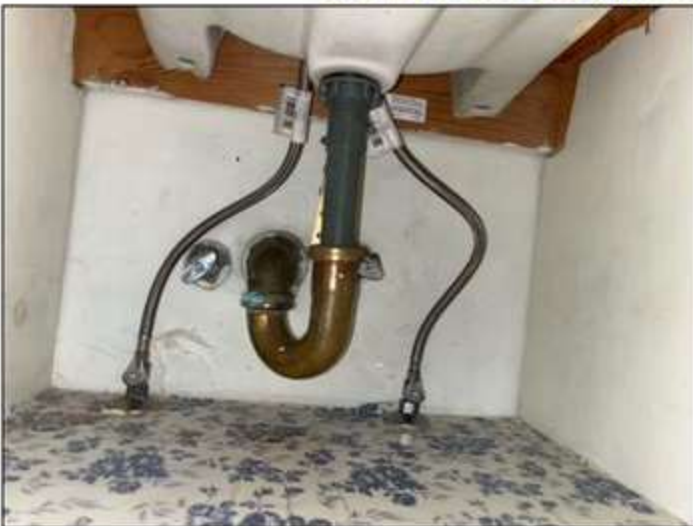
Bathroom (B) sink, sink faucet, and sink plumbing drain appear serviceable. Right side
