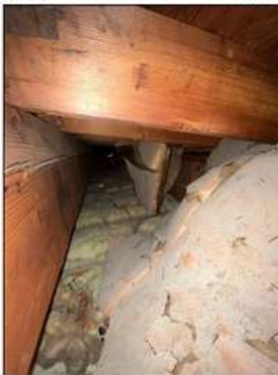
Attic structure is conventional wood framing 2x4 ceiling joist and 2x4 roof rafters, wood panel roof.
