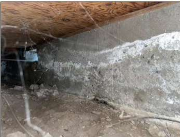
Raised foundation is poured concrete.
