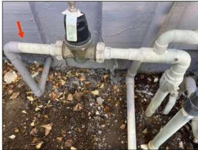
Pressure regulator installed at front of main water supply at meter area.
