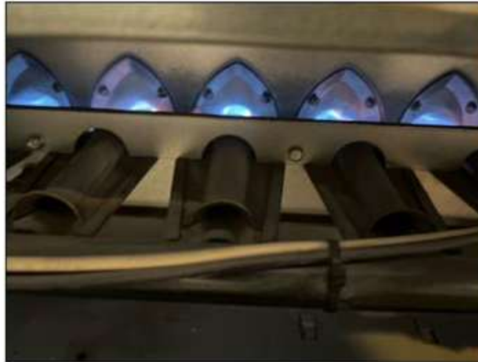
Furnace burner flame appears typical.
