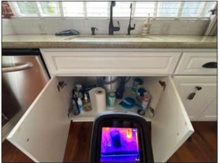
Thermal imaging was used to inspect interior of property, no visible abnormalities detected at the time of the inspection at this area.
