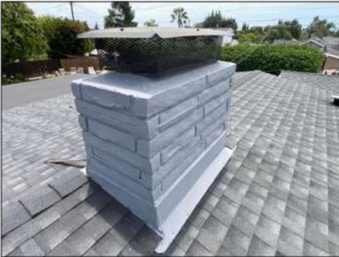
Chimney spark screen is installed, appears serviceable.
