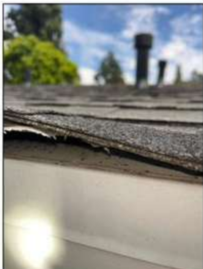
(one Layer) Main roof at area that was inspected has one layer of roof material installed.
