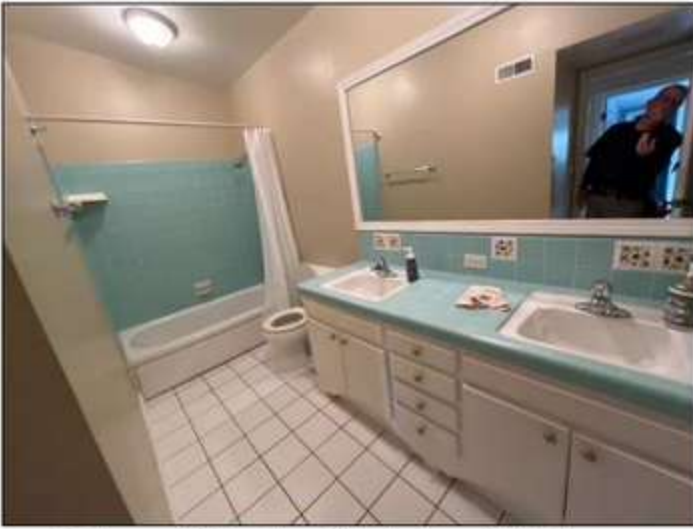
Bathroom (B) location: Main hallway full bathroom.
