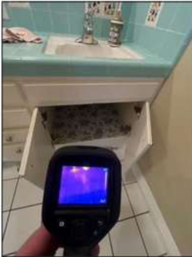
Thermal imaging was used to inspect interior of property, no visible abnormalities detected at the time of the inspection at this area.
