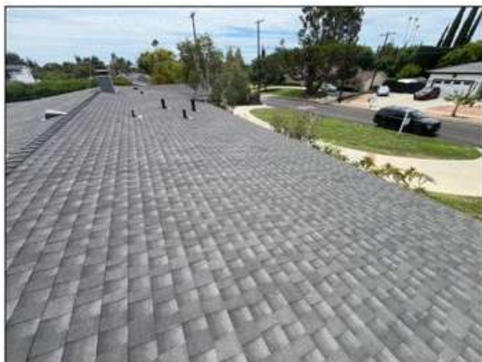
(W Face) Main roof on west face appears serviceable.
