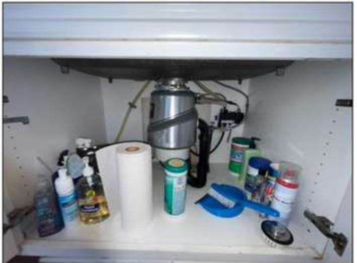
Plumbing under kitchen sink serviceable.
