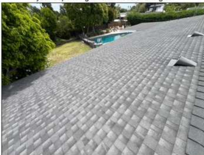
(E Face) Main roof on east face appears serviceable.
