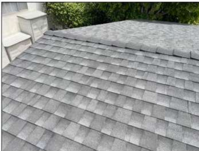
Roof installed at property: Asphalt composition architectural shingles installed at property, average life span 20 to 30 year depending on thickness of shingle.
